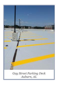
various repairs to the precast structural elements, extensive waterproofing (including traffic coating membrane over top deck and on stair tower floors), cleaning of the drainage system, and re-striping of the second and third levels.
